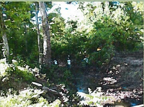
Workers collect debris at a previous NRCS' EWP site.
