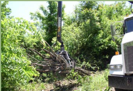
Debris removal from EWP project at Collinsville supervised by NRCS.
