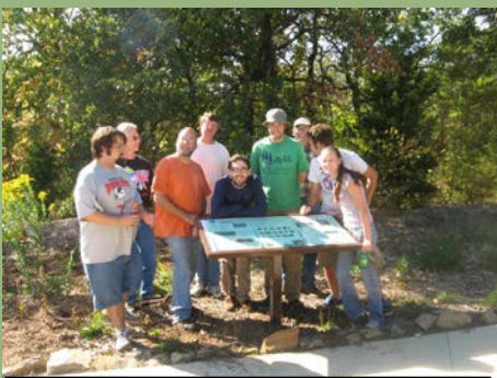
TCCD volunteers assisting with the installation of rain garden signage at Remington Elementary.
