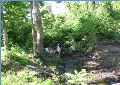
Workers collect debris at a previous NRCS' EWP site.
