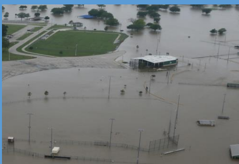
NRCS did not have any EWP's in Tulsa County, but due to torrential spring rains, Tulsa and surrounding areas had massive flooding.
