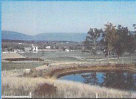
Pond construction has been one of the conservation practices included in the Conservation Cost Share Program.
